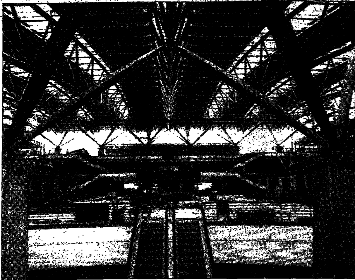
Enlarging Hamburg Airport: By the end of the decade, 12 million passengers a year will be handled.
